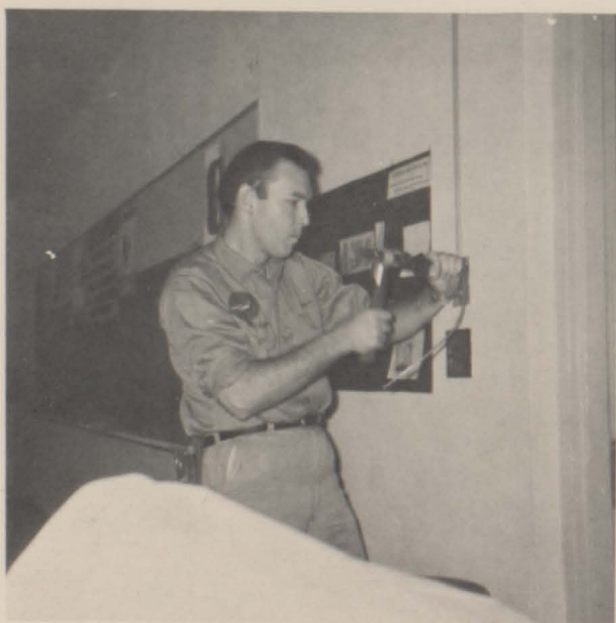
Installing a Switch Box for the Intercom System
