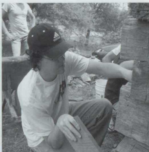
Above: Senior Kaleb Long concretes the cabin to seal the cracks. Right: Senior Will Vandergrift scrapes the last of the concrete out of the wheelbarrow.
